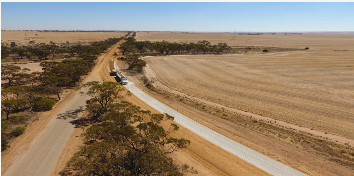
Cement stabilising underway on the Bruce Rock Narembeen Road
